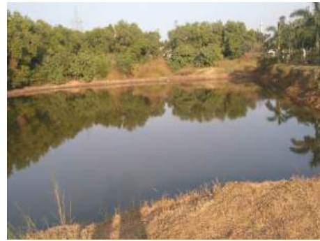
Rainwater harvesting pond after enhancement
